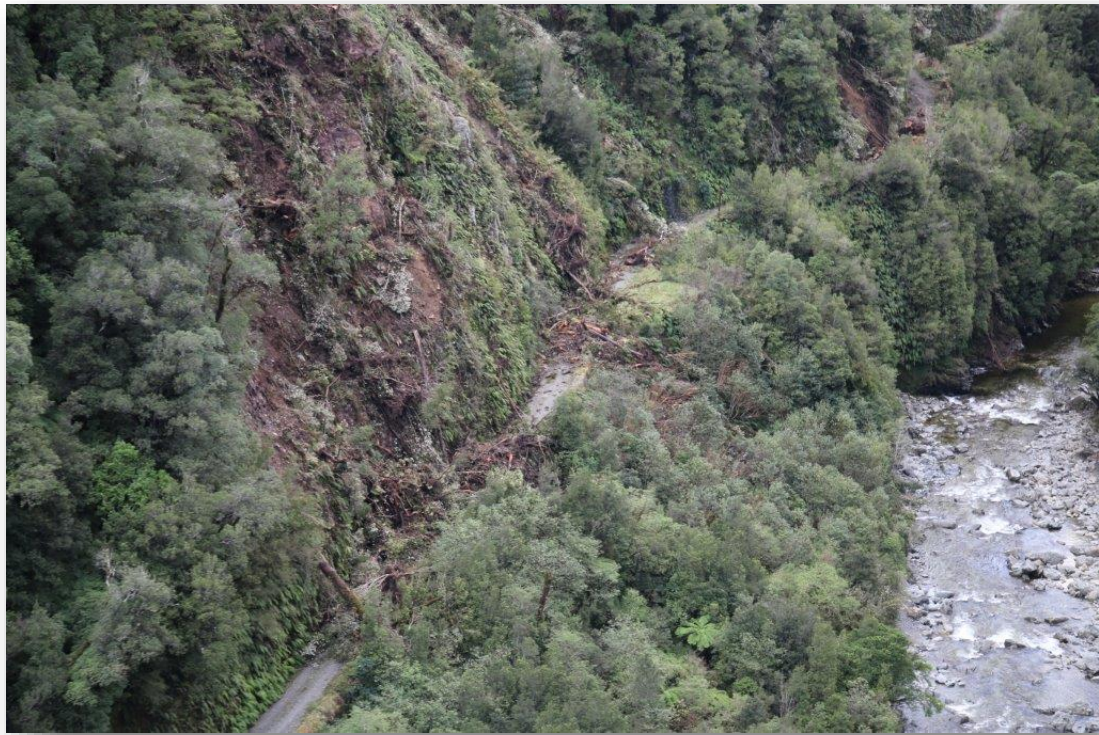
Road slip, South Westland.
