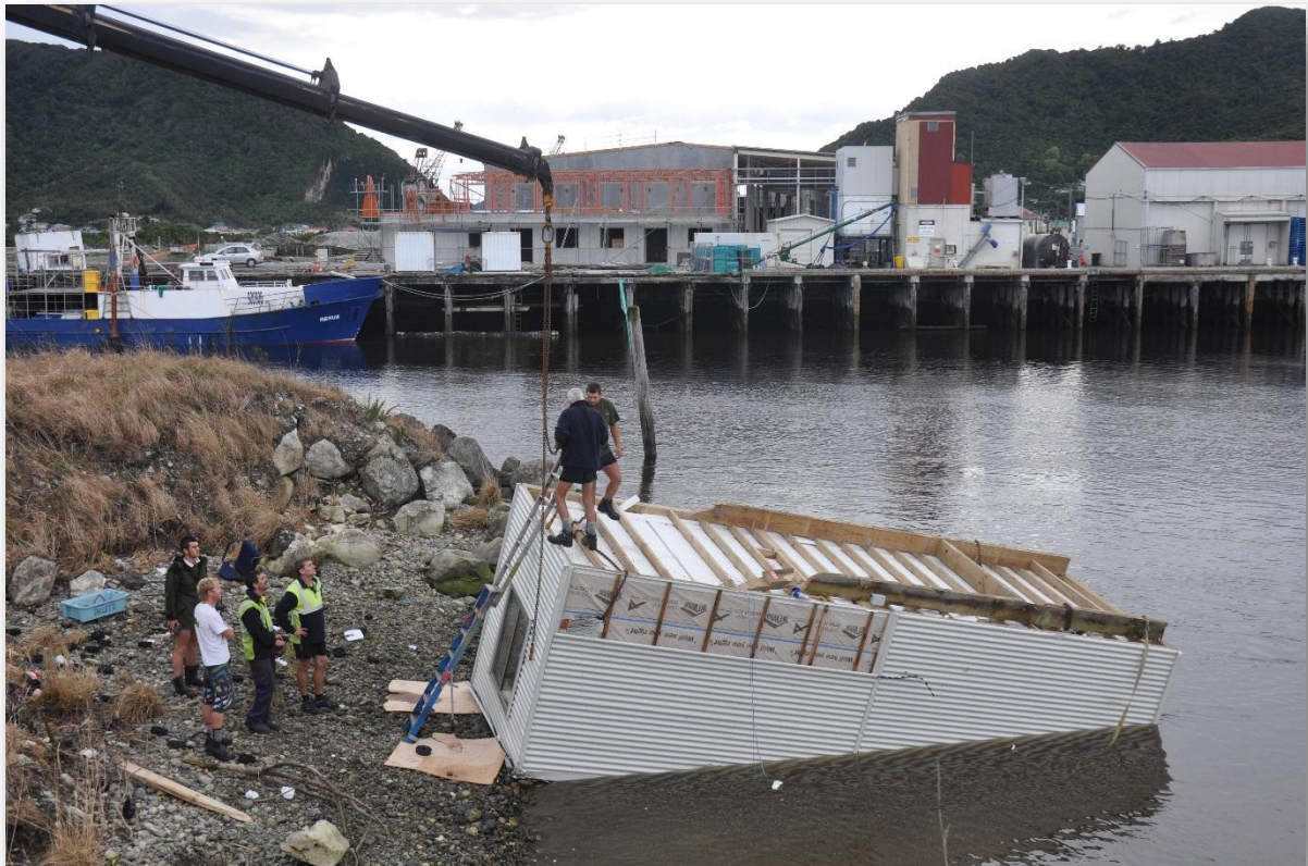
Westfleet site building blown into the Grey River.
