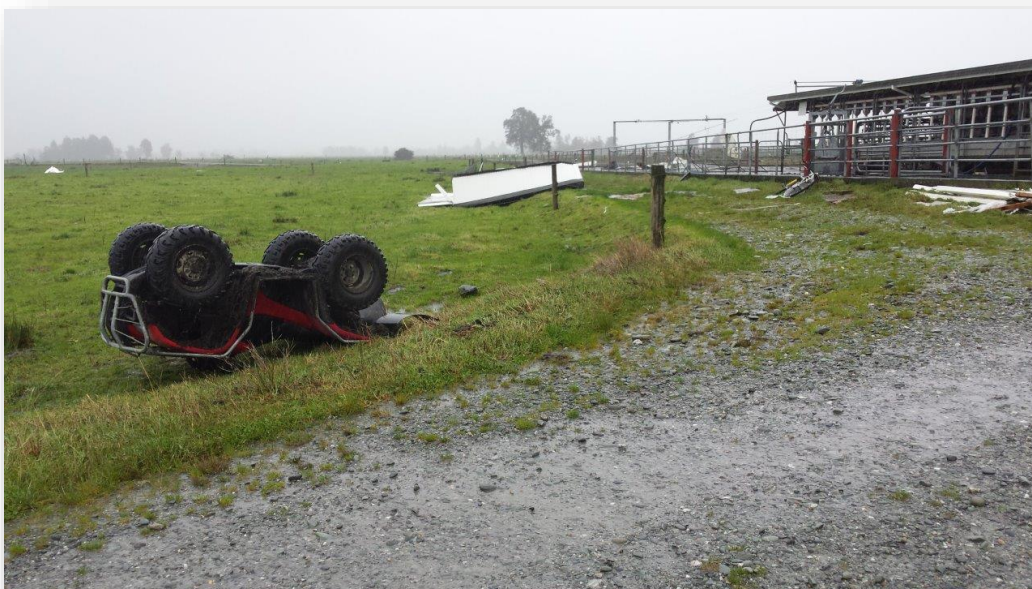
Damage to a dairy shed and farmbike.
